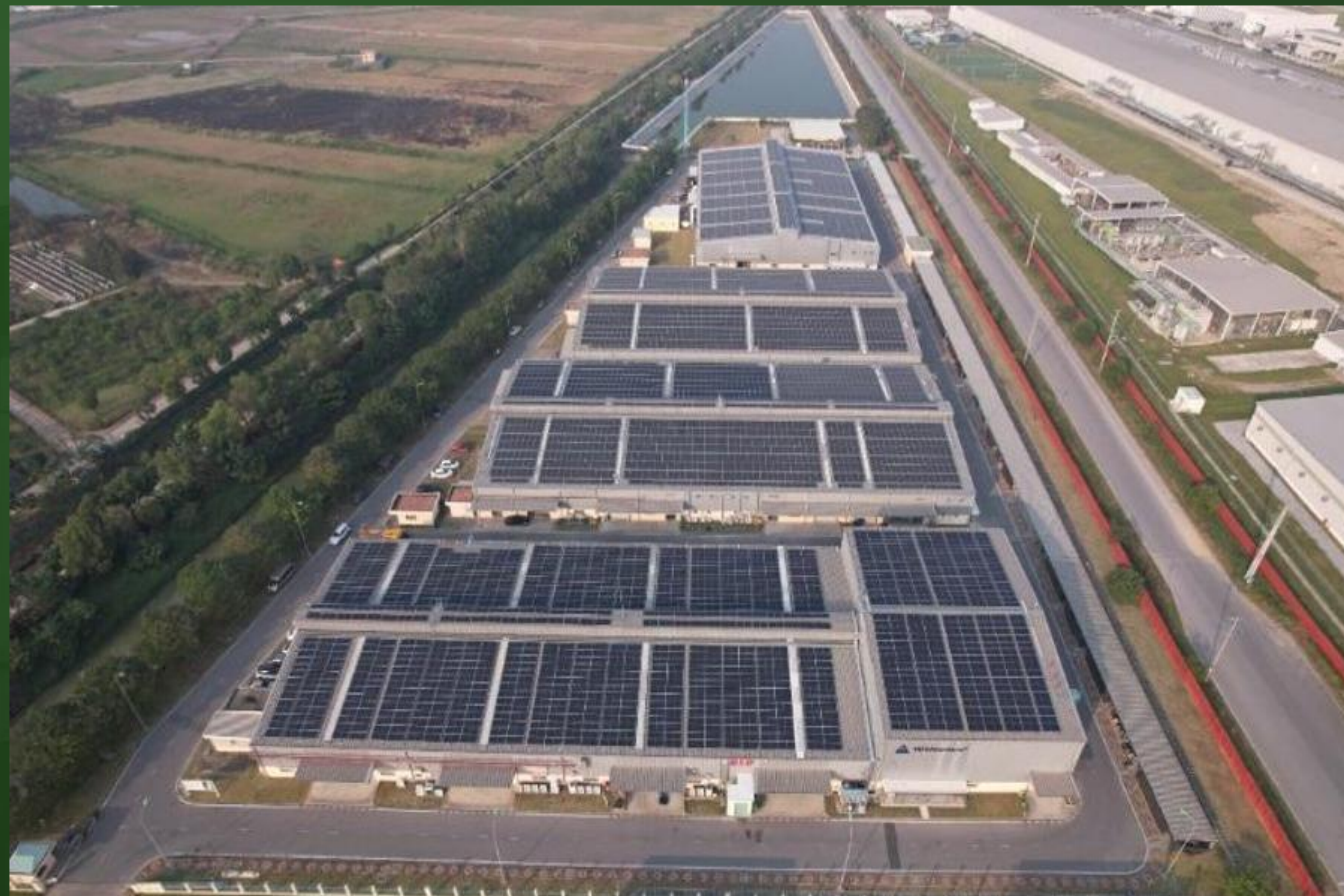
Rooftop Solar Project in Thang Long II Industrial Park Management
