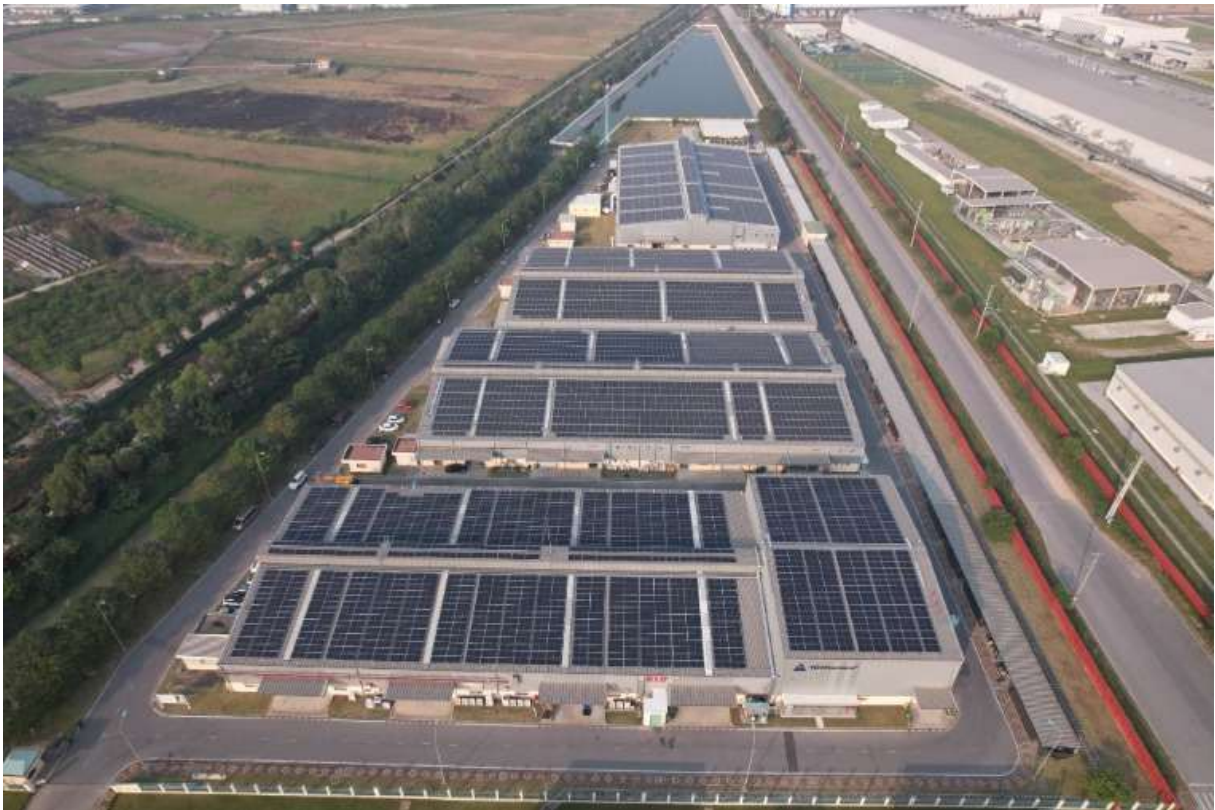
Figure 4-1: Rooftop Solar Project in Thang Long II Industrial Park Management Board
