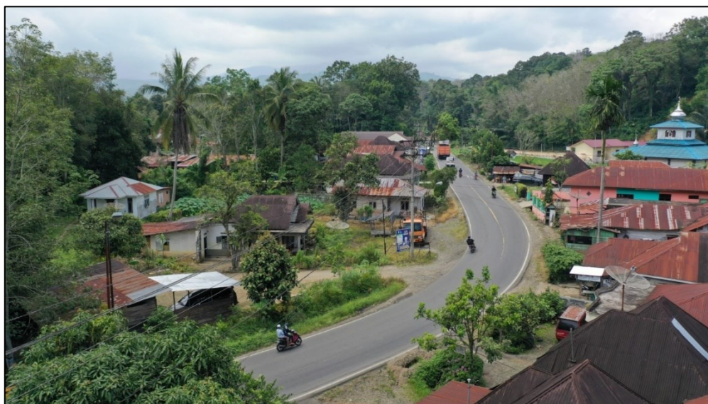
Figure 15. Typical road layout in rural Indonesia. Winding roads of ~6 to 7 m wide serving both local, regional, and national traffic. Overhead power and telecommunication cables with poles on both sides of the road. Buildings are in close proximity. Within cities and larger towns, the roads are generally slightly wider, but with more overhead cables, poles, and advertisement billboards.
