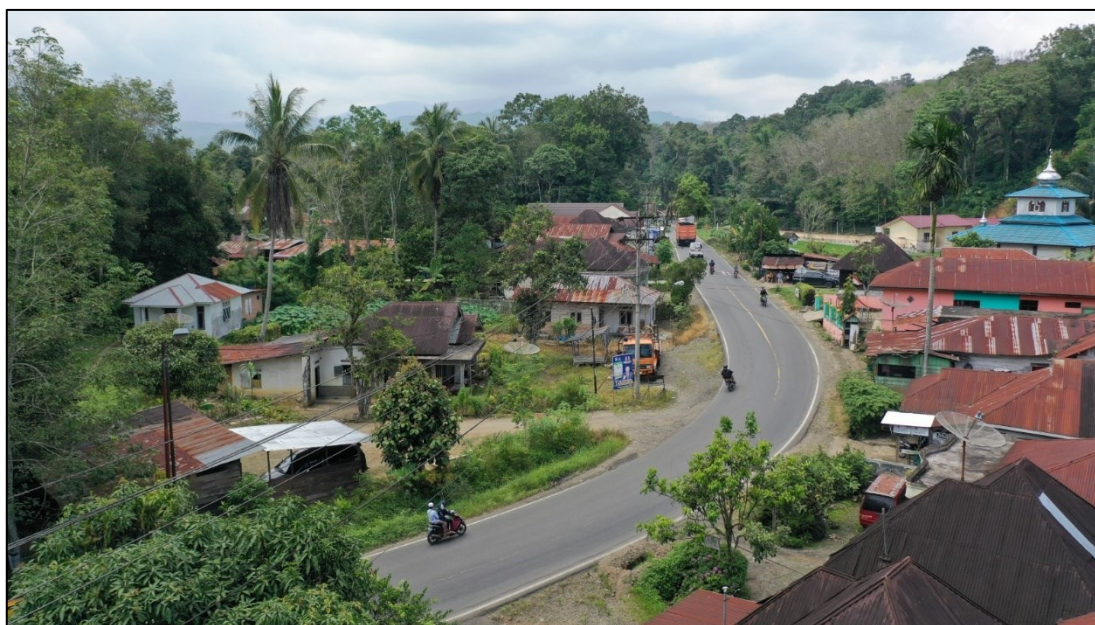
Figure 18. Typical road layout in rural Indonesia. Winding roads of ~6 to 7 m wide serving both local, regional, and national traffic. Overhead power and telecommunication cables with poles on both sides of the road. Buildings are in close proximity. Within cities and larger towns, the roads are generally slightly wider, but with more overhead cables, poles, and advertisement billboards.
