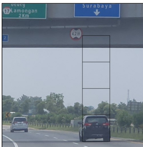
Figure 17. The height of bridges above road surface seems to be more than 4.2 m. As a comparison, this Toyota Innova Reborn's height is 1.795 m according to specifications.
