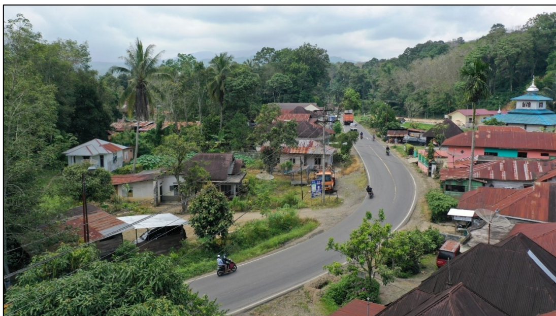
Figure 13. Typical road layout in rural Indonesia. Winding roads of ~6 to 7 m wide serving both local, regional, and national traffic. Overhead power- and telecommunication cables with poles on both sides of the road. Buildings are in close proximity. Within cities and larger towns, the roads are generally slightly wider, but with more overhead cables, poles, and advertisement billboards.
