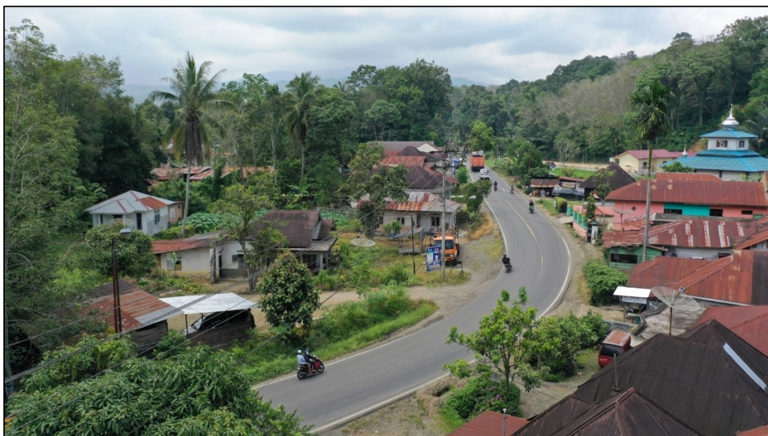
Figure 14. Typical road layout in rural Indonesia. Winding roads of ~6 to 7 m wide serving both local, regional, and national traffic. Overhead power- and telecommunication cables with poles on both sides of the road. Buildings are in close proximity. Within cities and larger towns, the roads are generally slightly wider, but with more overhead cables, poles, and advertisement billboards.
