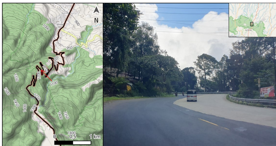
Figure 19. Section with hairpins south of Bandar Baru. In the sharp turns the road has been widened significantly.
